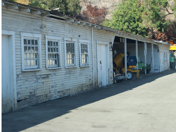
Figure 84: Nursery Garage and Maintenance Facility Building, 1927. Photo: ICF Jones & Stokes, August 2007
