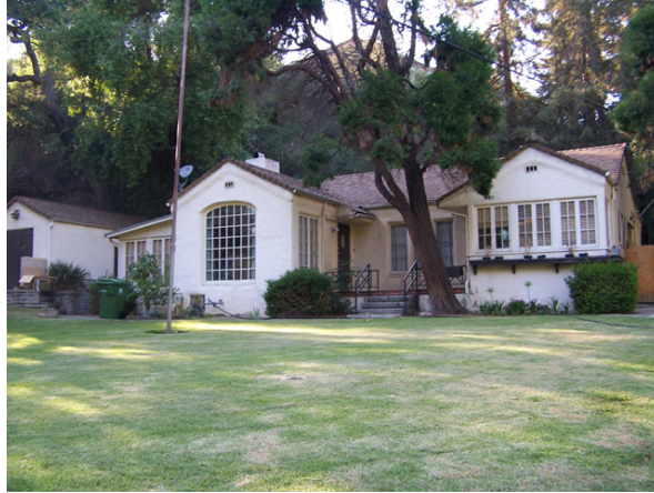
Figure 101: Fern Dell: Watchman's House and former Fern Dell Nature Museum, c.1927. View N. Photo: ICF Jones & Stokes, October 2007
