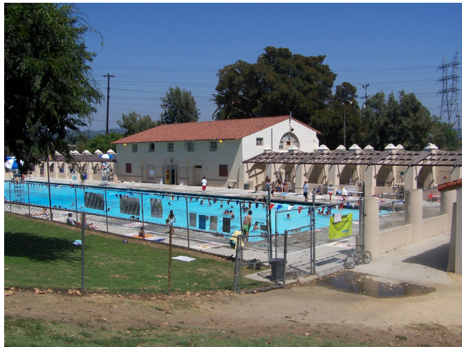
Figure 12: Griffith Park Recreation Center: Plunge and Poolhouse, 1927. View NE. Photo: ICF Jones & Stokes, August 2007
