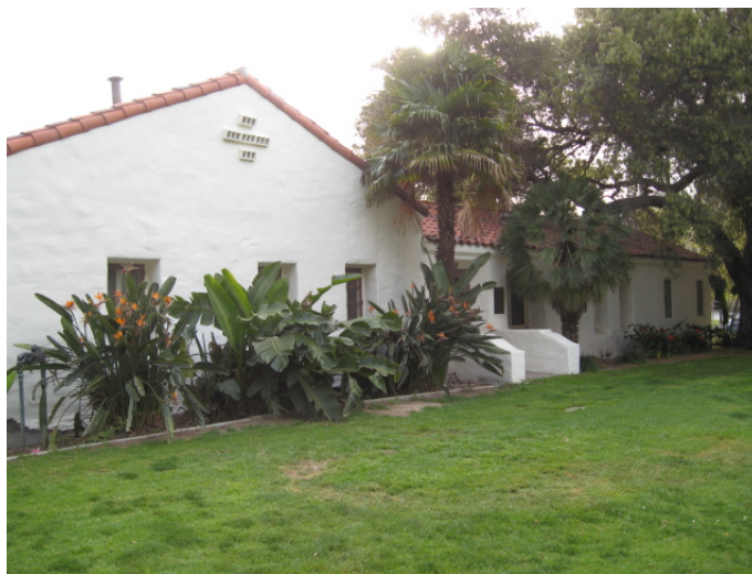
Figure 30: Feliz Adobe, 1853, exterior renovation in 1940s. View NE. Photo: ICF Jones & Stokes, March 2008.
