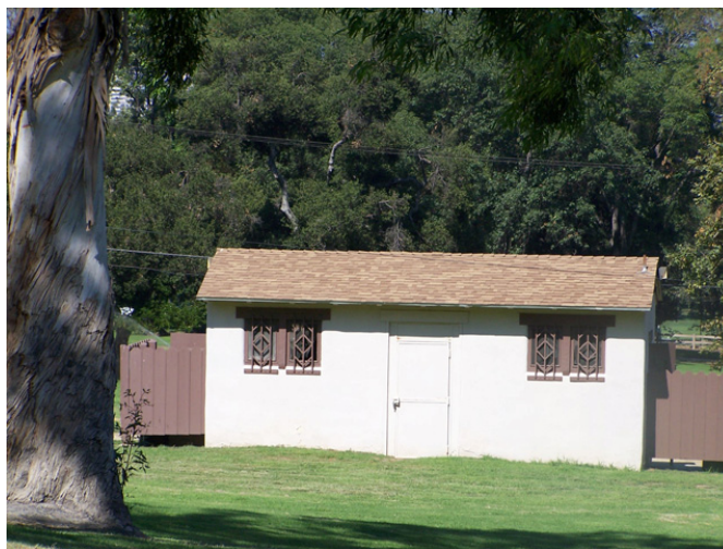
Figure 62: Park Center: Restroom Facility. View E. Photo: ICF Jones & Stokes, August 2007
