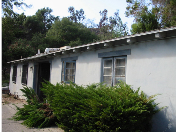
Figure 83: Nursery Office and Locker Room Building, 1927. Photo: ICF Jones & Stokes, October 2007
