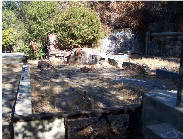
Figure 57: Foundation of Zoo Keepers House above the Old Zoo, c.1914. View SE. Photo: ICF Jones & Stokes, July 2007.
