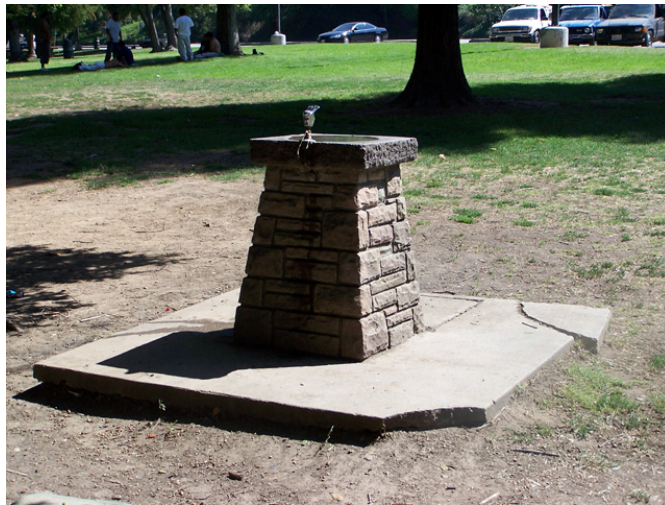
Figure 116: Ashlar cut drinking fountain near Pony Rides, c.1948. View SE. Photo: ICF Jones & Stokes, March 2008.
