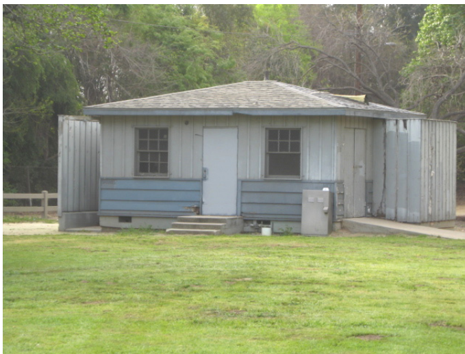
Figure 25: Restroom building, c.1948. View SE. Photo: ICF Jones & Stokes, March 2008.
