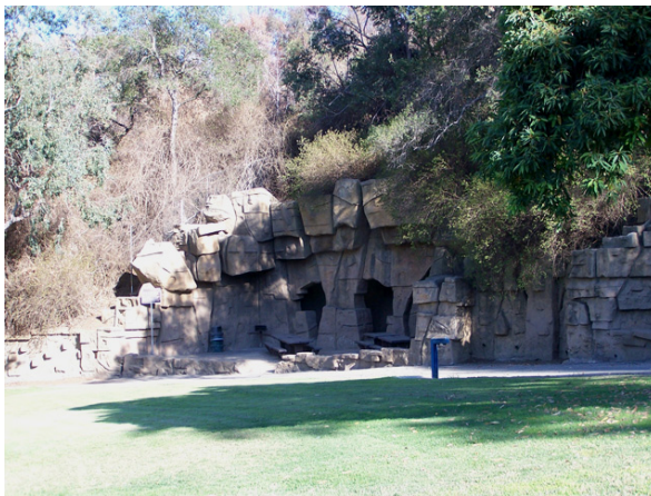
Figure 55: Old Zoo Picnic Area, Public Works Construction, c. 1932. View SW. Photo: ICF Jones & Stokes, July 2007.
