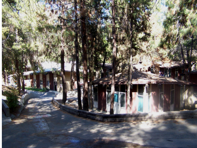
Figure 52: Griffith Park Boys Camp. View E. Photo: ICF Jones & Stokes, August 2007.
