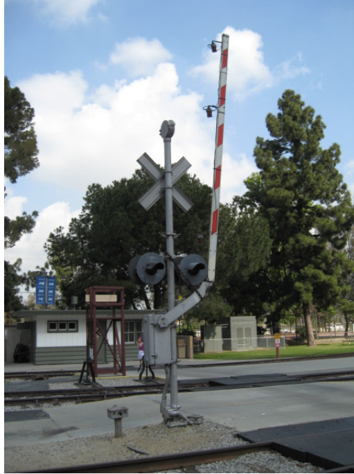
Figure 46: Train signal with 1952 administrative building in background. Travel Town Transportation Museum. View NE. Photo: ICF Jones & Stokes, March 2008.
