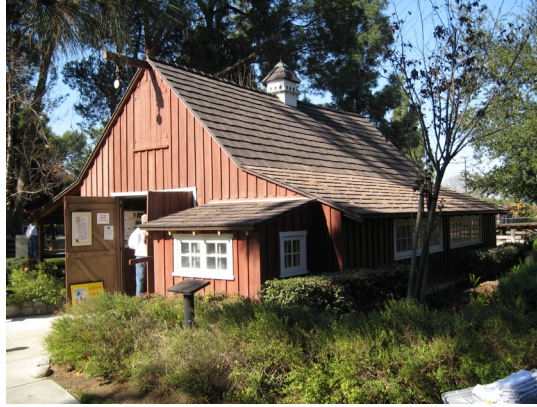
"Walt's Barn," 1950. Built by Disney Studio Architect John Kowles Jr. Los Angeles Live Steamers Railroad Museum. Photo: ICF Jones & Stokes, January, 2008
