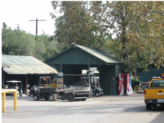
Figure 59: Service Station within Turf Maintenance Facility View S. Photo: ICF Jones & Stokes, October 2007
