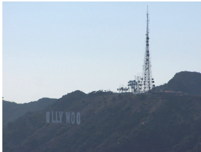
Figure 123: Mt. Lee Radio Towers, Hollywood Sign. View N. Photo: ICF Jones & Stokes, October 2007.
