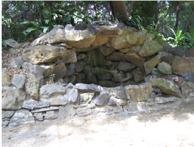
Figure 94: Fern Dell detail. View NW. Photo: ICF Jones & Stokes, March 2008.
