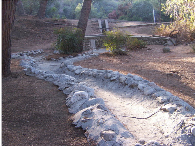
Figure 114: Drainage element near Greek Theatre picnic area, c.1935. View W. Photo: ICF Jones & Stokes, March 2008.
