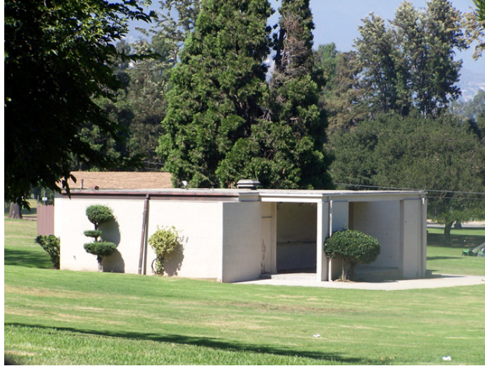
Figure 61: Park Center: Seal Show Building, 1954. View NW. Photo: ICF Jones & Stokes, August 2007
