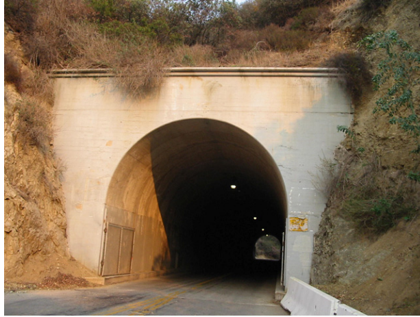
Figure 89: Mt. Hollywood Tunnel. View E. Photo: ICF Jones & Stokes, October 2007
