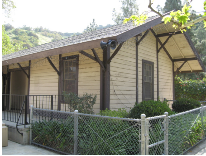
Figure 45: Depot, Travel Town Transportation Museum. View SE. Photo: ICF Jones & Stokes, March 2008.
