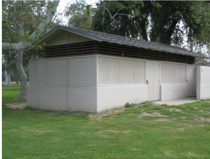
Figure 27: Crystal Springs Picnic Area restroom structure, c. 1951. View NE. Photo: ICF Jones & Stokes, March 2008.
