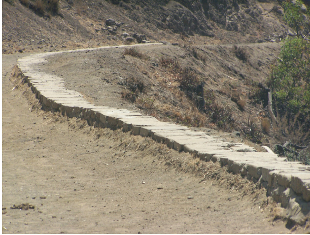
Figure 107: Recycled concrete boundary leading to Bronson Caves. View S. Photo: ICF Jones & Stokes, March 2008.
