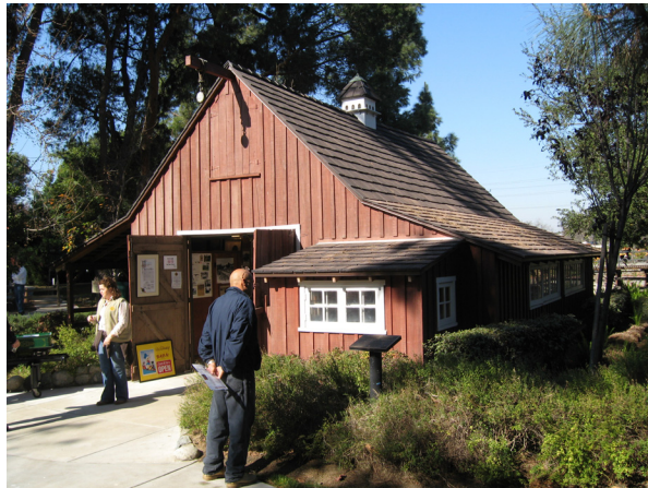
Figure 41: “Walt’s Barn,” 1950. Los Angeles Live Steamers Railroad Museum. View NW. Photo: ICF Jones & Stokes, January 2008
