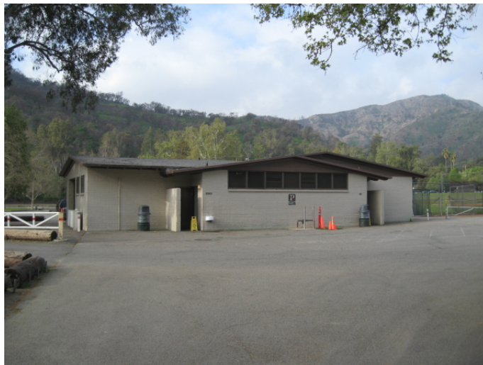
Figure 29: Field House and Comfort Station, 1951. View SW. Photo: ICF Jones & Stokes, March 2008.
