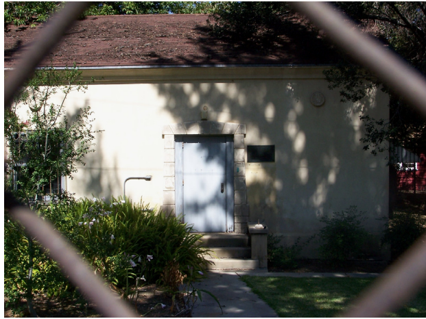
Figure 23: Los Angeles City Infrastructure Building. View E. Photo: ICF Jones & Stokes, August 2007
