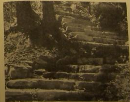
Wheeler Dam Reservation, Tennessee Valley Authority
